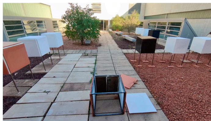
Figure 1. Aspect of the sample cubes during construction.
